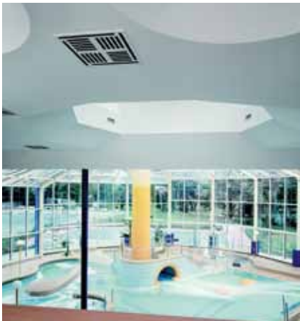
Ceiling with acoustic lining in an indoor swimming pool
