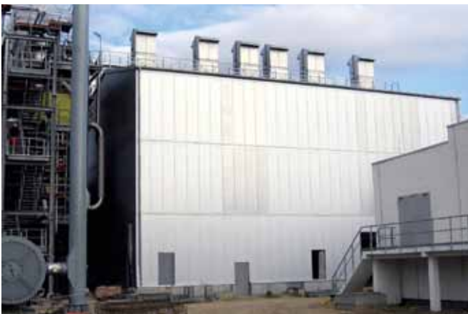
Hall construction with sound insulation
