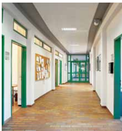
Corridor ceiling lining F30, hinged
