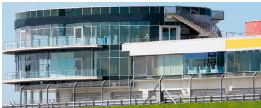
Post-girt construction for a circular building
