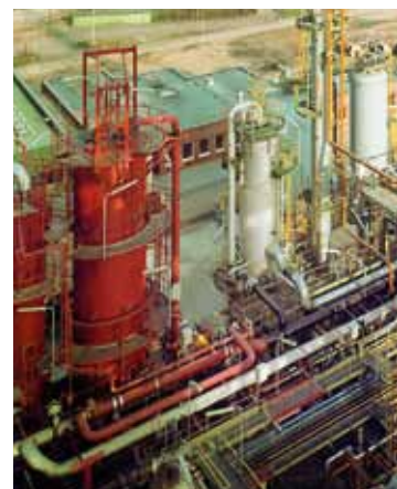
Corrosion protection of columns and pipes
