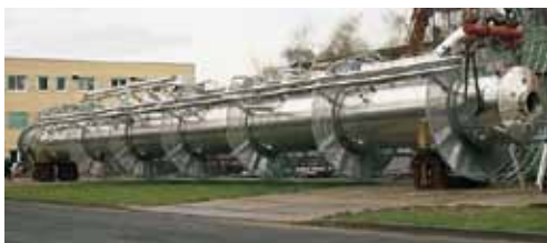
Insulation work on columns
