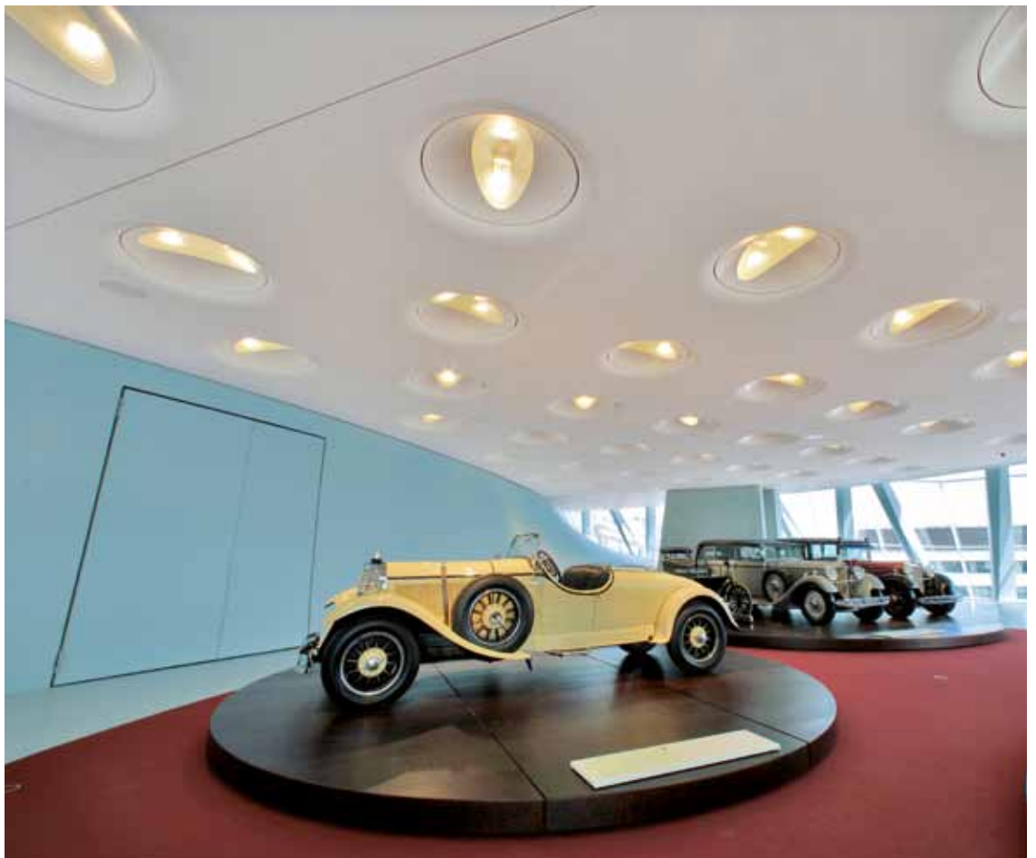
Perforated plaster ceiling with integral special lamps
