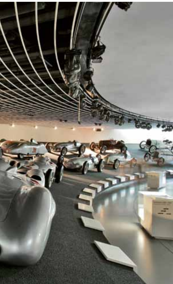
Ceiling composed of tubular lamellae in a museum
