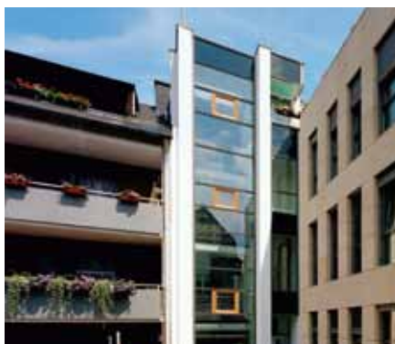
Girt-girt-structure in a staircase and aluminium window with vertical sun protection louvers
