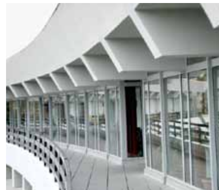
Room-high glass façade elements with polygonal arrangement in a circular building
