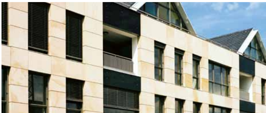
Aluminium window elements in a natural stone façade
