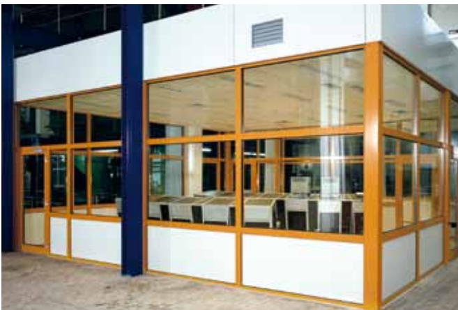
Switch room with air conditioning
