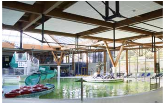
Suspended acoustic ceiling in an indoor swimming pool
